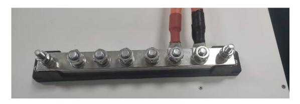
5. Afterwards, fix the main power cable: remove the flat washer, spring washer, nut 1, and nut 2 from the M8 screw on one end of the busbar.
