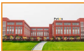
Shandong PYTES New Energy Technology
